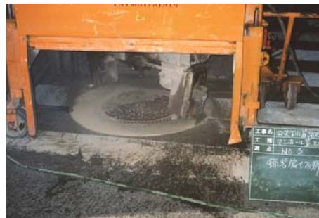
Rotating two-blade cutting wheel
